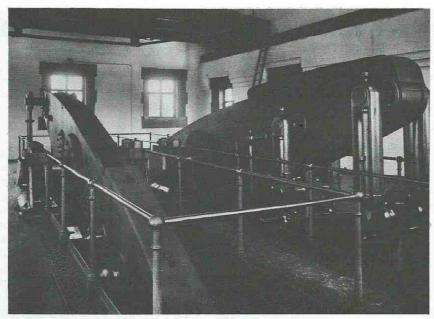
Beams of the Watt engine at Chelvey,
